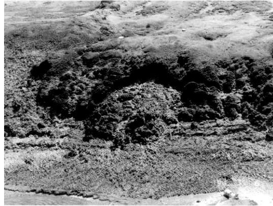
Figure 5 : Salt leaching and slope failure of case 2
